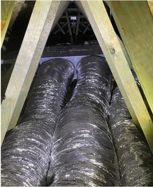
Distribution entirely outside the conditioned envelope
