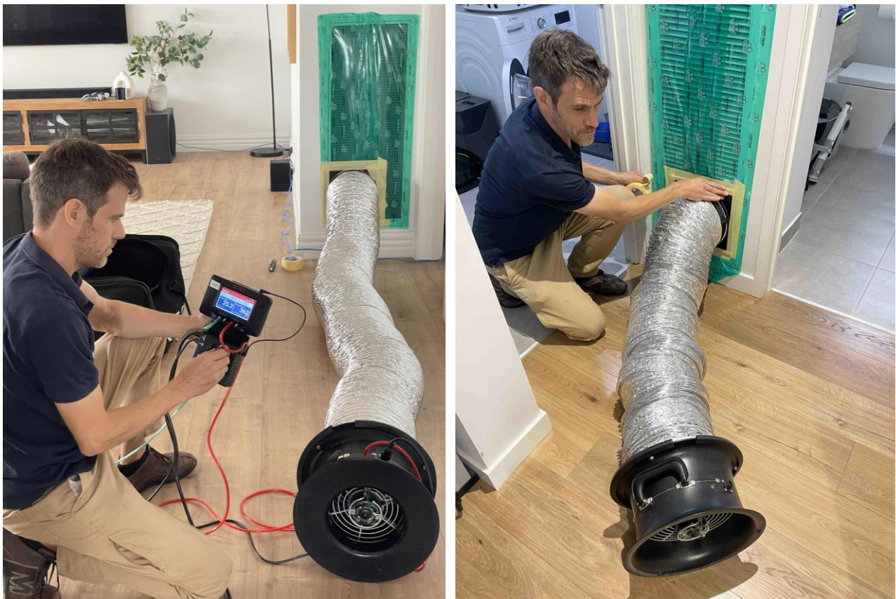
Figure 36 Duct testing setup
