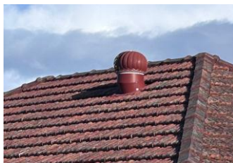
Figure 9.2 - Wind driven roof space ventilator
