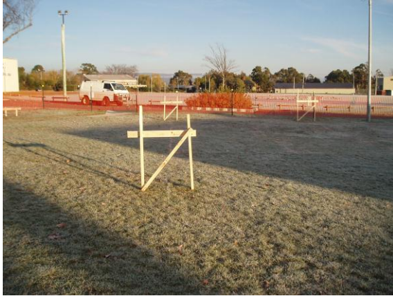
Figure 2.8 - Exclusion fence and commencement of site set out (June 5, 2006)
