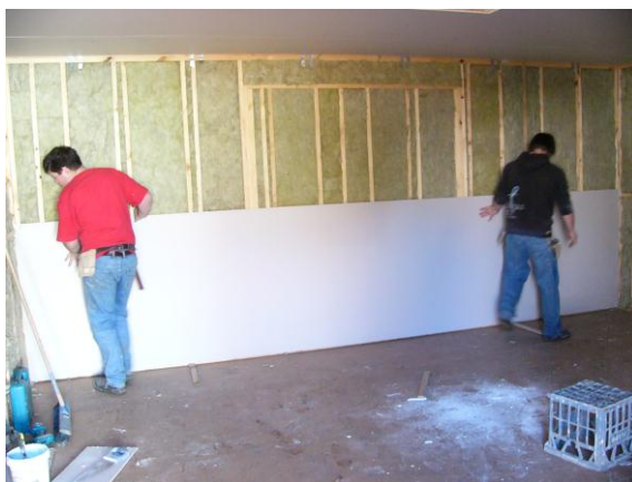
Figure 2.17 - Application of paper-faced gypsum plasterboard to walls (July 6, 2006)
