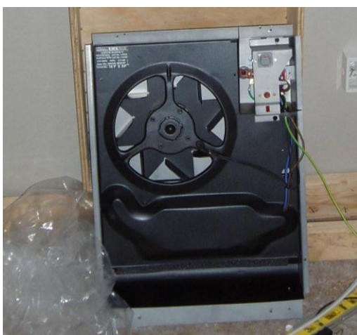
Figure 3.57 – Wall heater being installed during test cell construction
