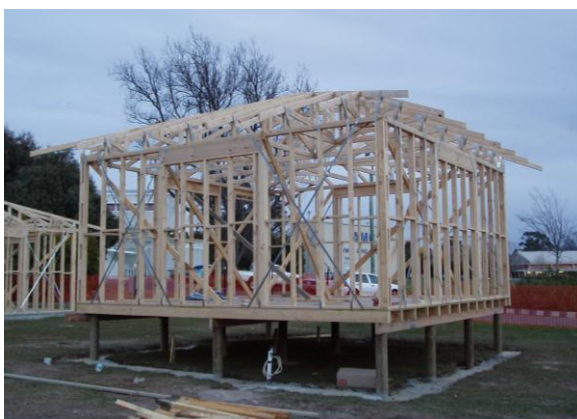
Figure 2.12 - Roof trusses erected on test cell (June 21, 2006)
