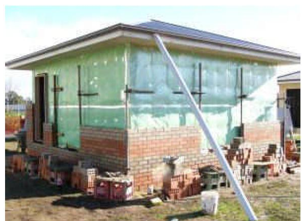
Figure 2.18 - Bricklaying well underway (July 6, 2006)
