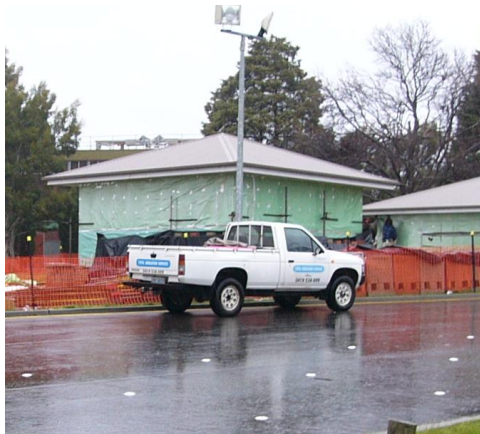
Figure 2.15 - Another rainy day halts external works (July 5, 2006)
