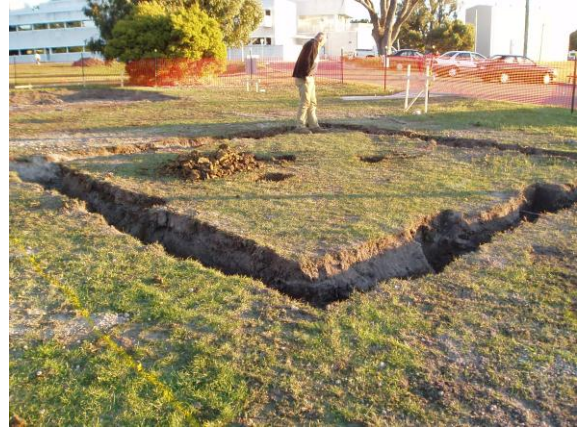
Figure 2.9 - Excavation for footings of test cell (June 7, 2006)
