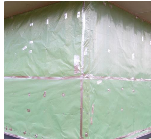
Figure 2.28 - Reflective foil tape repairs to building wrap during construction
