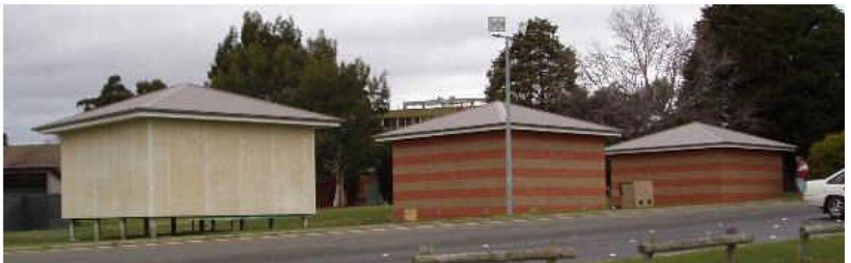
Figure 2.21 – The thermal performance test cells after site cleaning and removal of safety fence (July 15, 2006)
