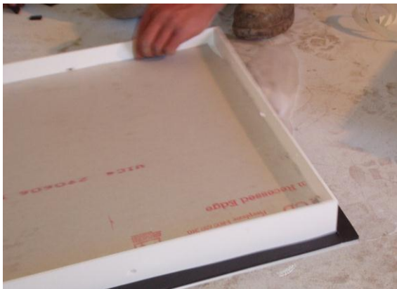
Figure 2.40 - Application of high density foam rubber tape to prefabricated insert
