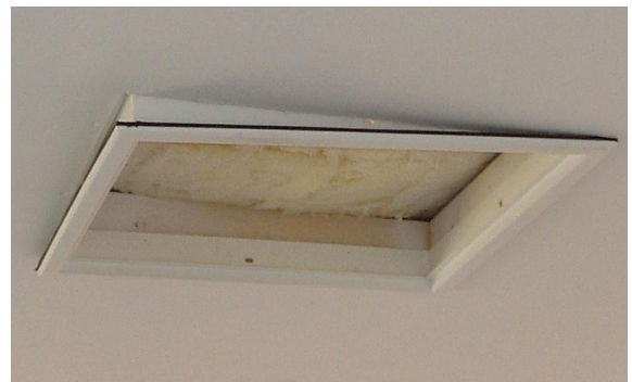
Figure 2.41 - Pushing prefabricated insert hard-up against the plasterboard ceiling
