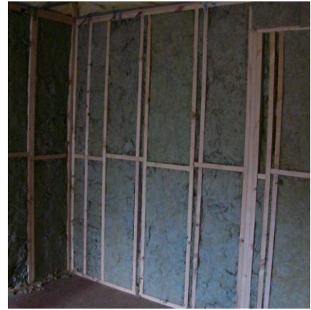
Figure 2.14 - Rockwool wall batt insulation (July 5, 2006)
