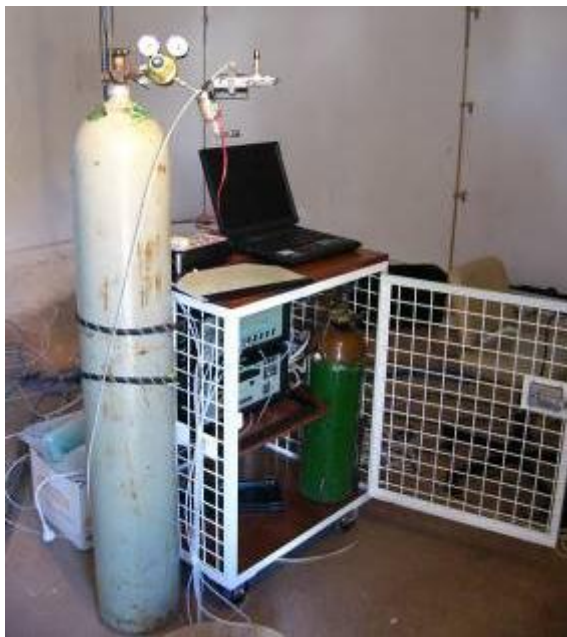
Figure 3.31 – SF 6 and CO 2 cylinders with Tracer gas equipment, which controlled gas dosing and measured gas decay in the test cell zones
