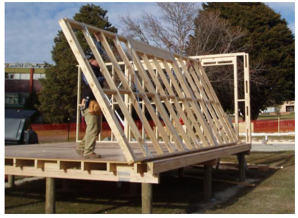
Figure 2.11 - The two-man process stage of erecting the prefabricated wall frames (June 20, 2006)
