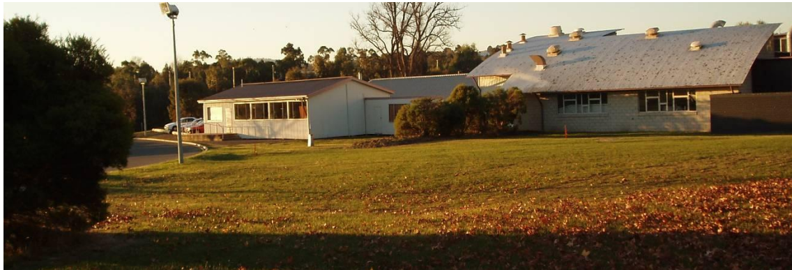
Figure 2.2 – Northern aspect of site
