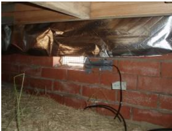
Figure 3.23 - Airflow measurement through the subfloor air vent of the test cell
