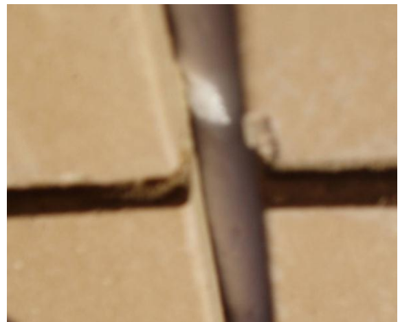
Figure 2.45 - Close up view of polypropylene rod inserted into construction joint
