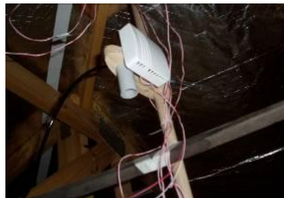
Figure 3.12 – Mid-roof space air temperature and relative humidity
