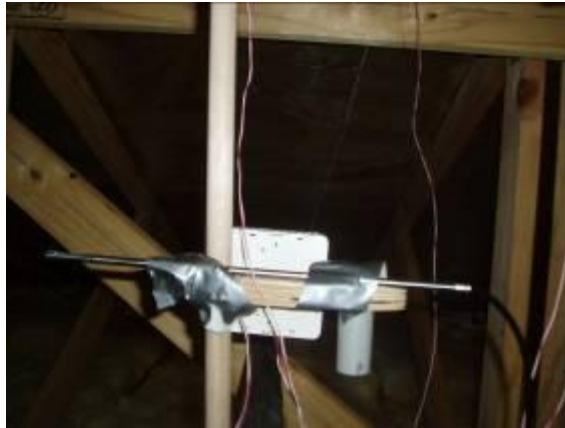
Figure 3.22 – Roof space vertical airflow measurement
