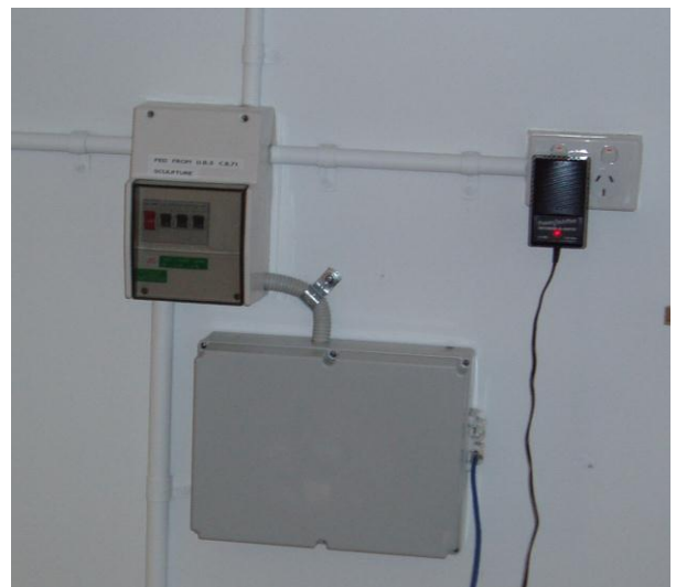
Figure 2.36 - Surface mounted electrical services when finished
