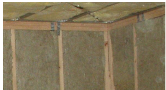
Figure 2.55 - Double top plate
