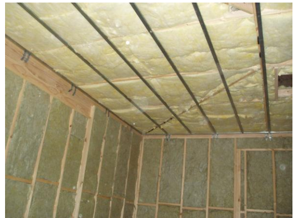
Figure 2.16 - Glasswool ceiling batt insulation installed (July 6, 2006)
