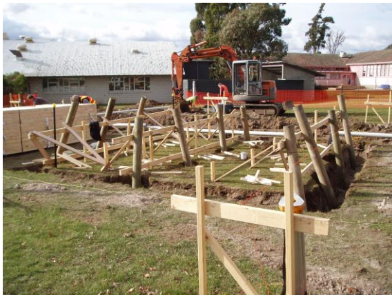
Figure 2.10 - Poles in place before concrete put in footings (June 13, 2006)
