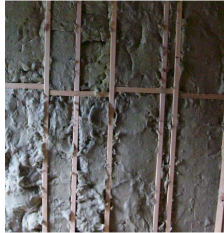
Figure 2.53 - Insulation installation in test cell 1 – third attempt
