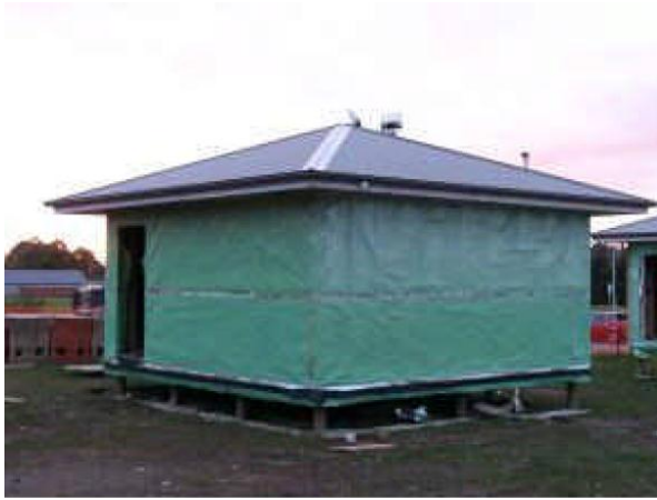
Completion of wall wrap and sheet metal roofing (July 3, 2006)
