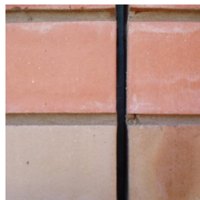
Figure 2.47 - External flexible sealant in construction joint
