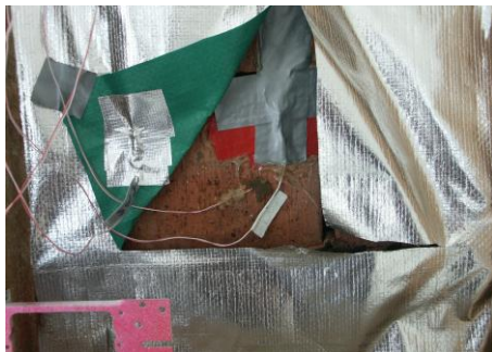
Figure 3.26 – Sensor attached to the outside surface of the building wrap
