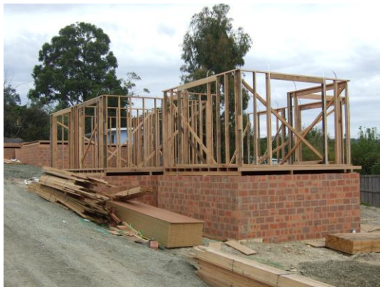
Figure 4.3 - Completed wall-framing stage of one of the platform floored houses
