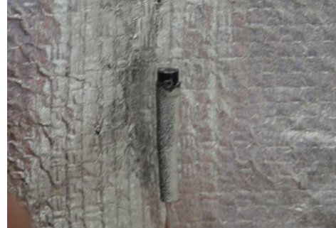
Figure 3.20 - Temperature sensor taped onto inside surface of roof sarking
