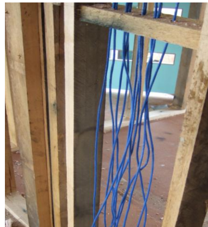
Figure 3.41 - Installation of data cables in hallway wall
