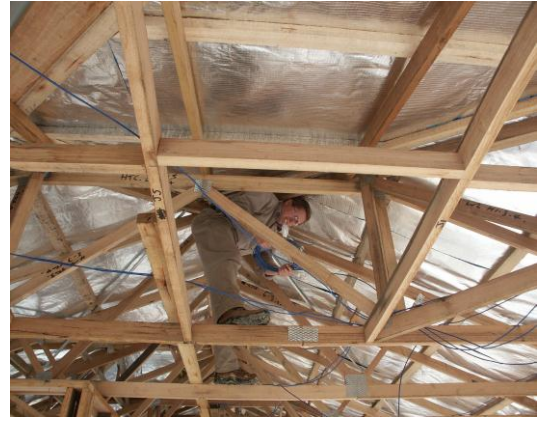
Figure 2.15 - Interior view of the roof trusses and reflective sarking
