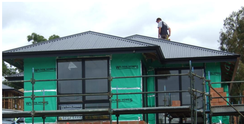
Figure 2.8 - Taping of building wrap at the case study house
