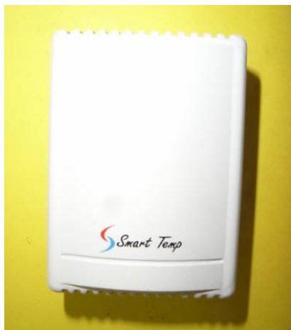
Figure 3.15 - Wall-mounted air temperature sensor located in a thermostat housing
