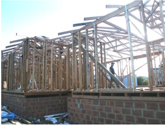
Figure 2.14 - Installation of timber roof trusses onto the exterior stud wall
