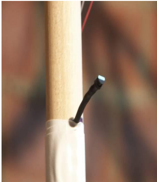
Figure 3.18 - Temperature sensor fixed to pole at mid roof space
