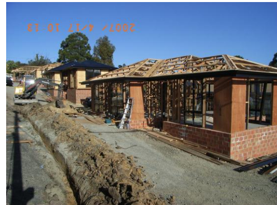
Figure 4.4 - Framing stage of the concrete slab test house
