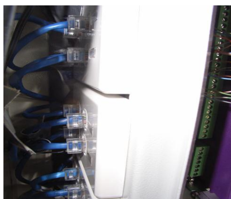
Figure 3.45 - Data cable and RJ 45 plugs connecting the data logger's RJ 45 terminals
