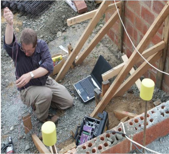
Figure 3.50 - Connecting and checking sensor feeder cable on site
